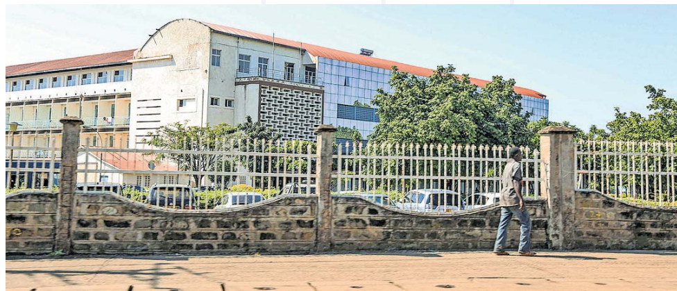
The Jaramogi Oginga Odinga Teaching and Referral Hospital in Kisumu, which was funded by the Russian government.
