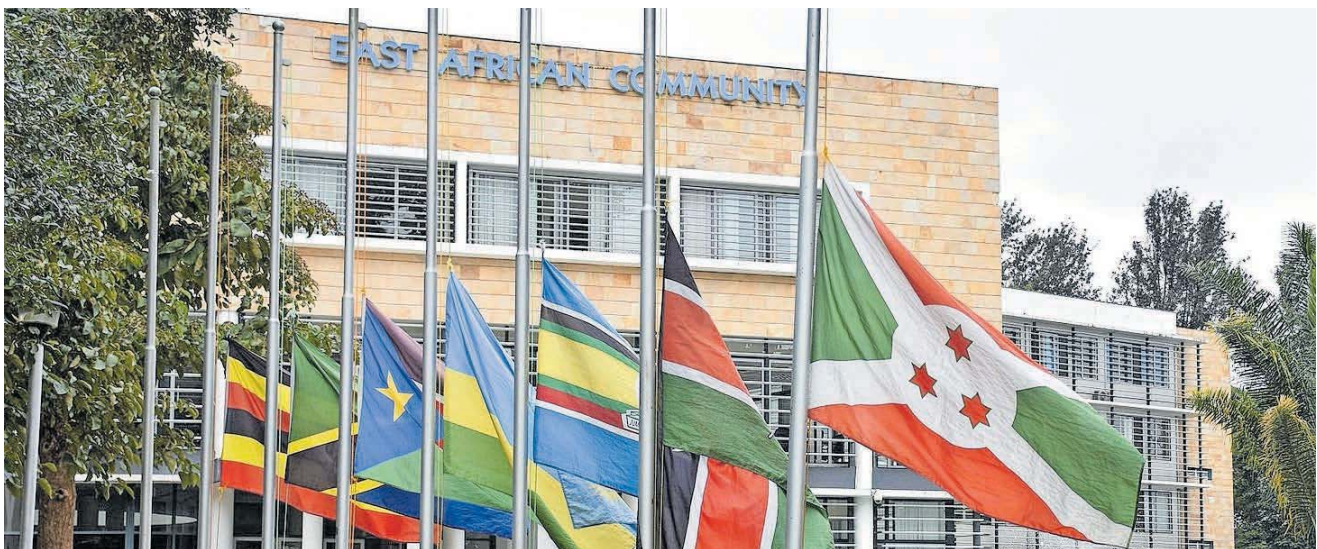
The East Africa Community headquarters in Arusha, Tanzania.
