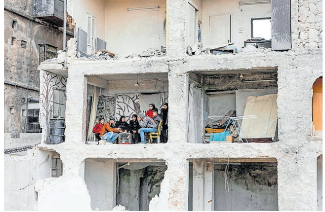
Ali al-Bash and his mother, Amina, drink coffee at home in a building damaged by the 7.8-magnitude quake in Aleppo city, Syria, on February 21. Once a major commercial hub, Aleppo had been battered by over a decade of war when the quake struck early this month. PHOTO | AFP
